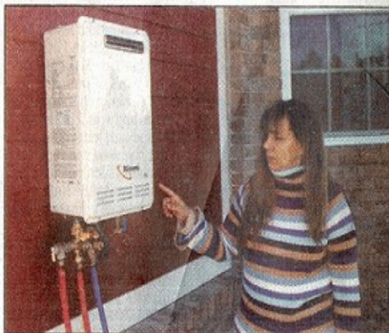
Alan Mauldin/Times-Enterprise Marlene Bienes displays the tankless water heater which provides hot water on demand without continuously heating water in a tank.
